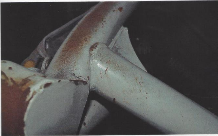
Fig. 7 — This top corner of the safety cage was subjected to significant force. The welds are flat to convex and held without failure during the crash.
